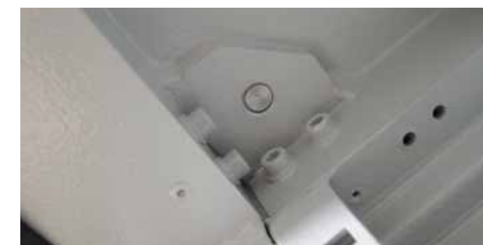
→ Riveted and welded cabinet frame - top
