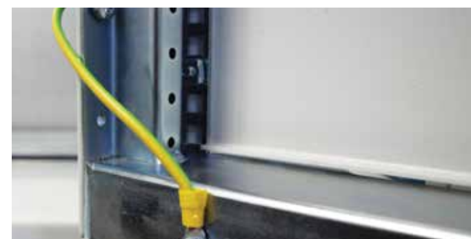
→ Earthing of the swing frame
