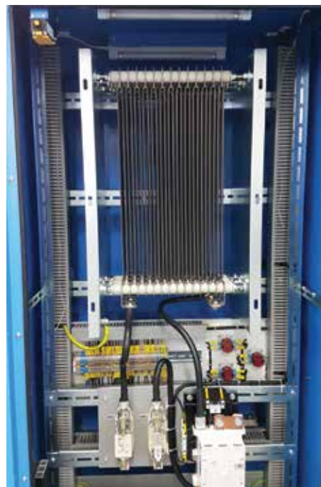
→ Installation of the AACE resistor in the FS-1-1 cable cabinet
