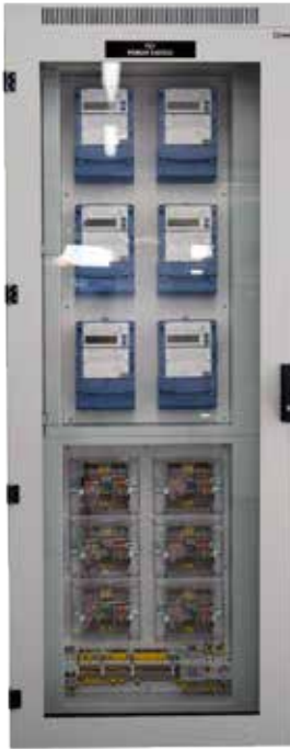
■ Metering cabinet with a mounted meter plate (swinging and fixed)
