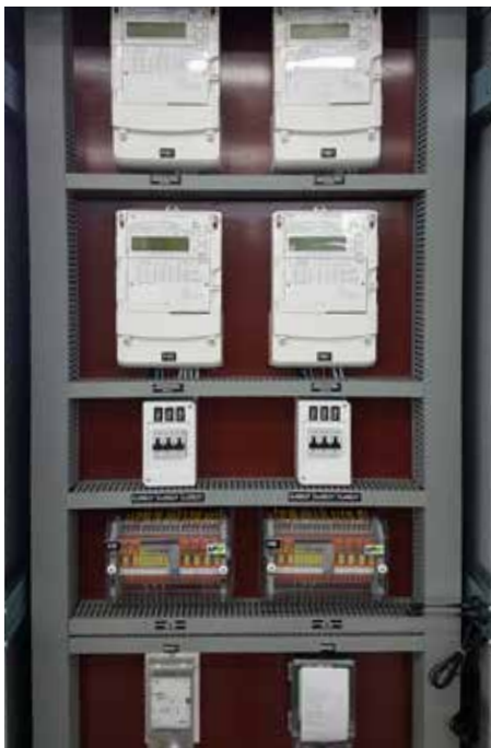
→ Mounting on a solid dielectric plate
