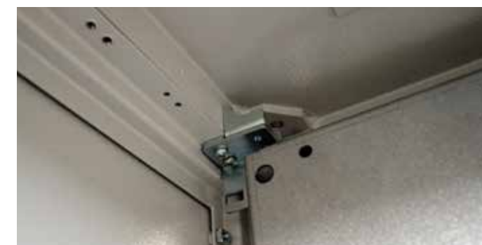
→ Mounting plate fixing elements
