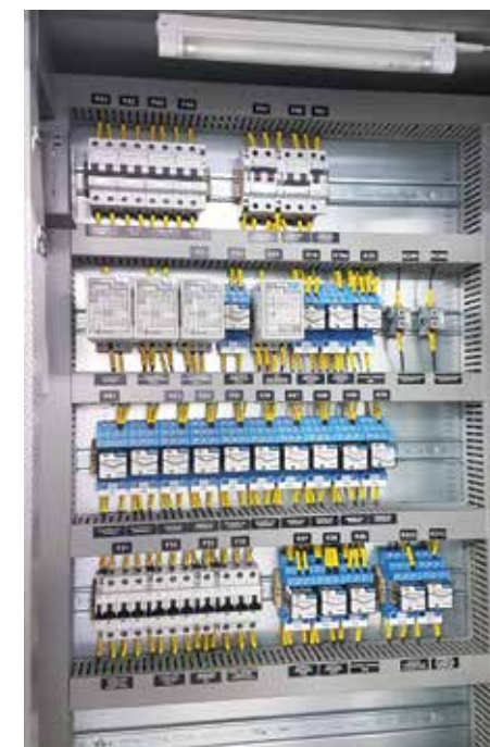
→ Installation of relays on the cabinet mounting plate
